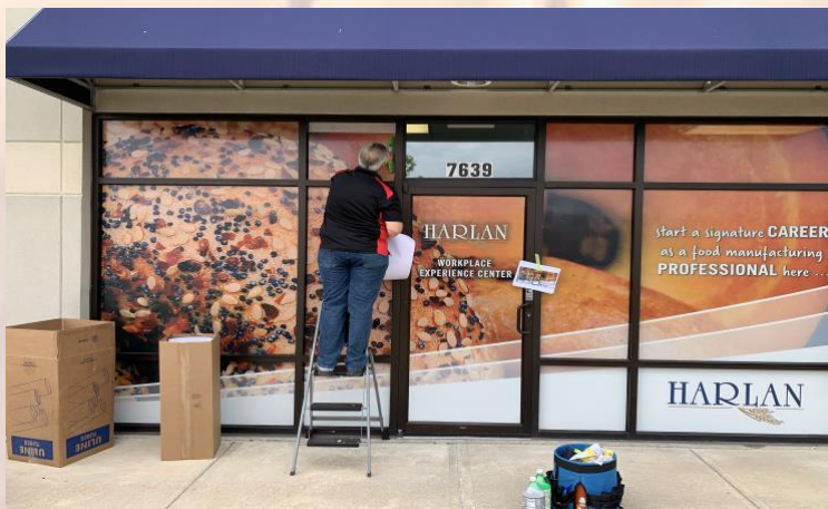
SAFE Workplace Simulation window clings being installed in Avon.
